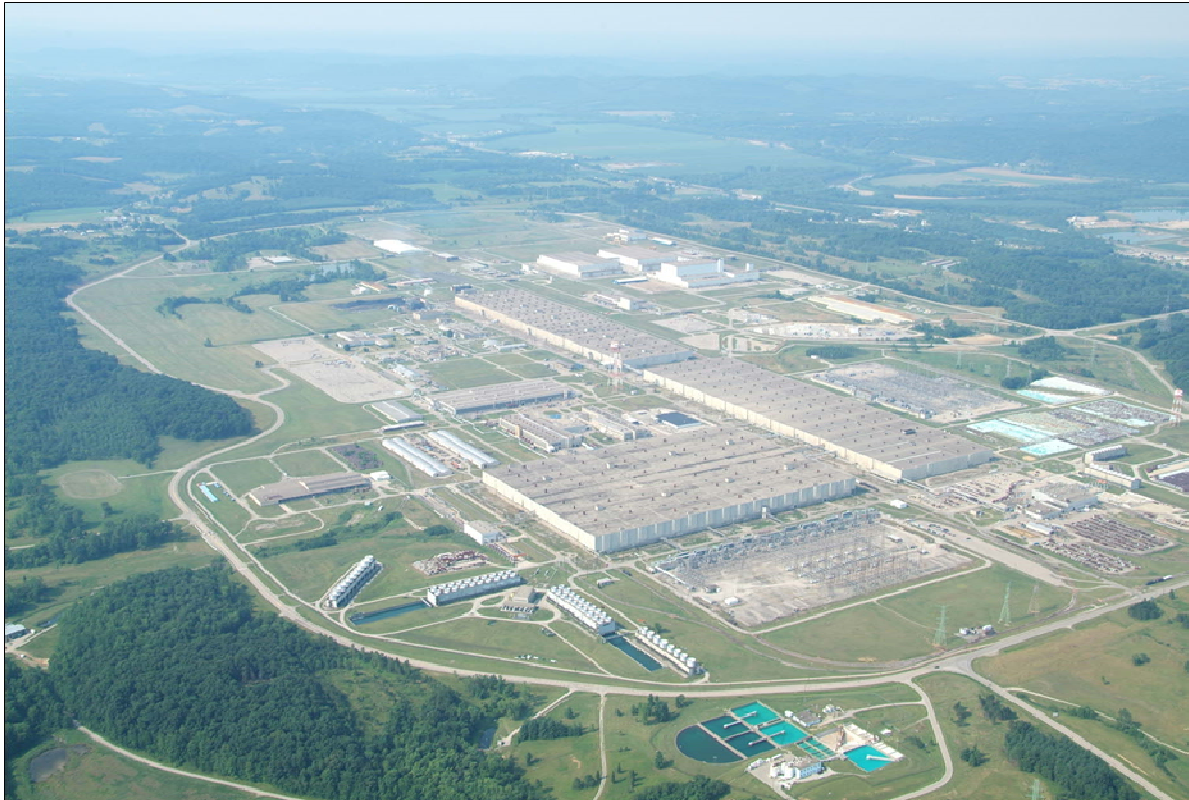
Figure 2. Aerial View of PORTS (circa early 2000s)
