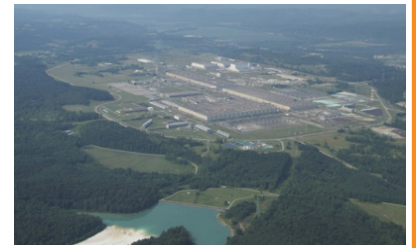
Photo: US Department of Energy (DOE)
